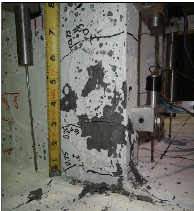
Figure 4-23: Spalled Region of the UHPC Pile Due to Crushing during the UPAC-2 Test after Completing of the 1.0-in. Load Displacement Cycles
