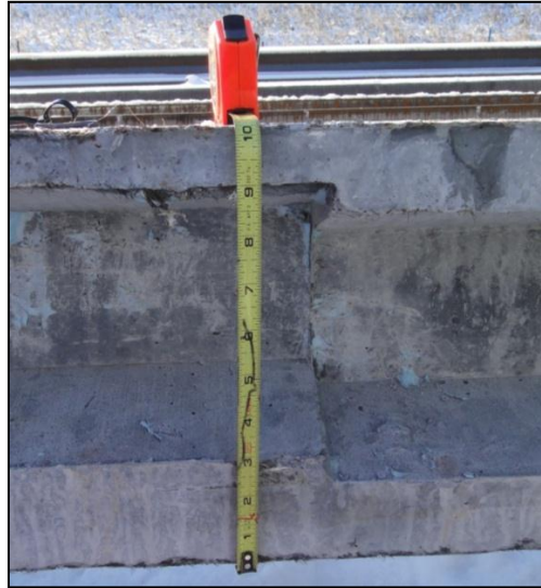
Figure 5-17: Change in the Flange Thickness of P3
