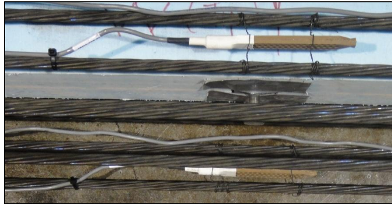
Figure D-3: Strung Embedded Concrete Strain Gage
