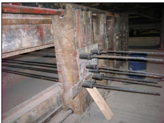
Figure 4-8: Prestressing Strands Layout at the Anchorage end
