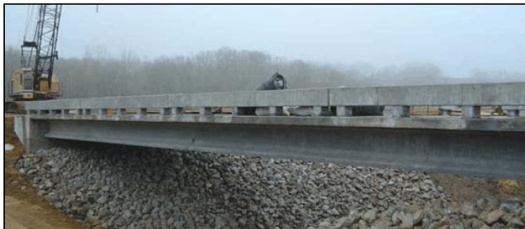
Figure 2-4: The UHPC Girder Bridge in Wapello County, Iowa (Wipf 2009)
