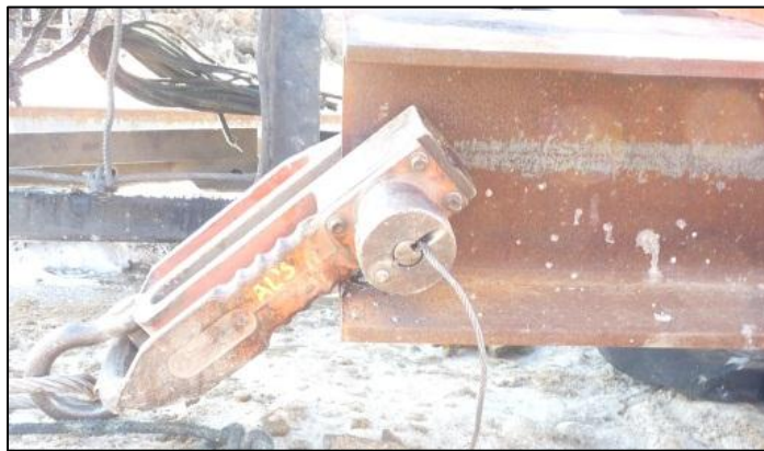
Figure 6-17: Steel HP 10 x 57 Production Pile Pickup Point
