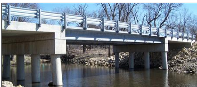
Figure 2-7: Jakway Park Bridge in Iowa using PI-Girders (FHWA 2011)
