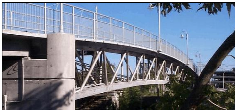
Figure 2-3: Sherbrooke Pedestrian Bridge, Quebec, Canada (Ductal 2012)
