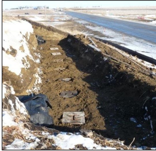
Figure 6-16: Layout of Abutment Piles
