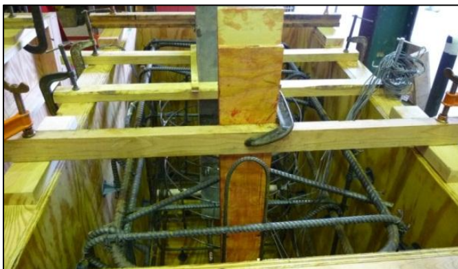
Figure 4-10: Abutment Cap Steel Reinforcement Inside of Forms
