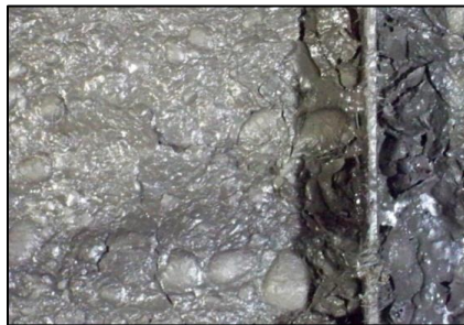
Figure 5-15: Clumps in UHPC after Batching for the 11/21/2011 Pour
