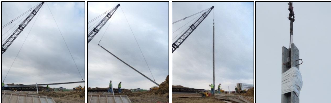
Figure 6-18: Stages in Lifting UW1-2
