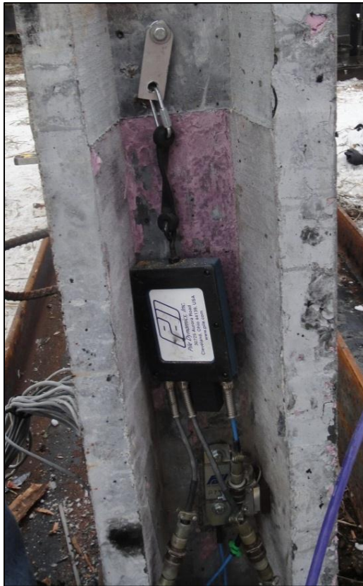
Figure 5-28: Attached PDA Equipment during the Installation of P3
